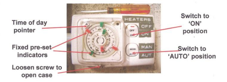
The Space Heating Time Clock controls the water pump that pumps the hot water to the heaters in the bedrooms and the main living area.
